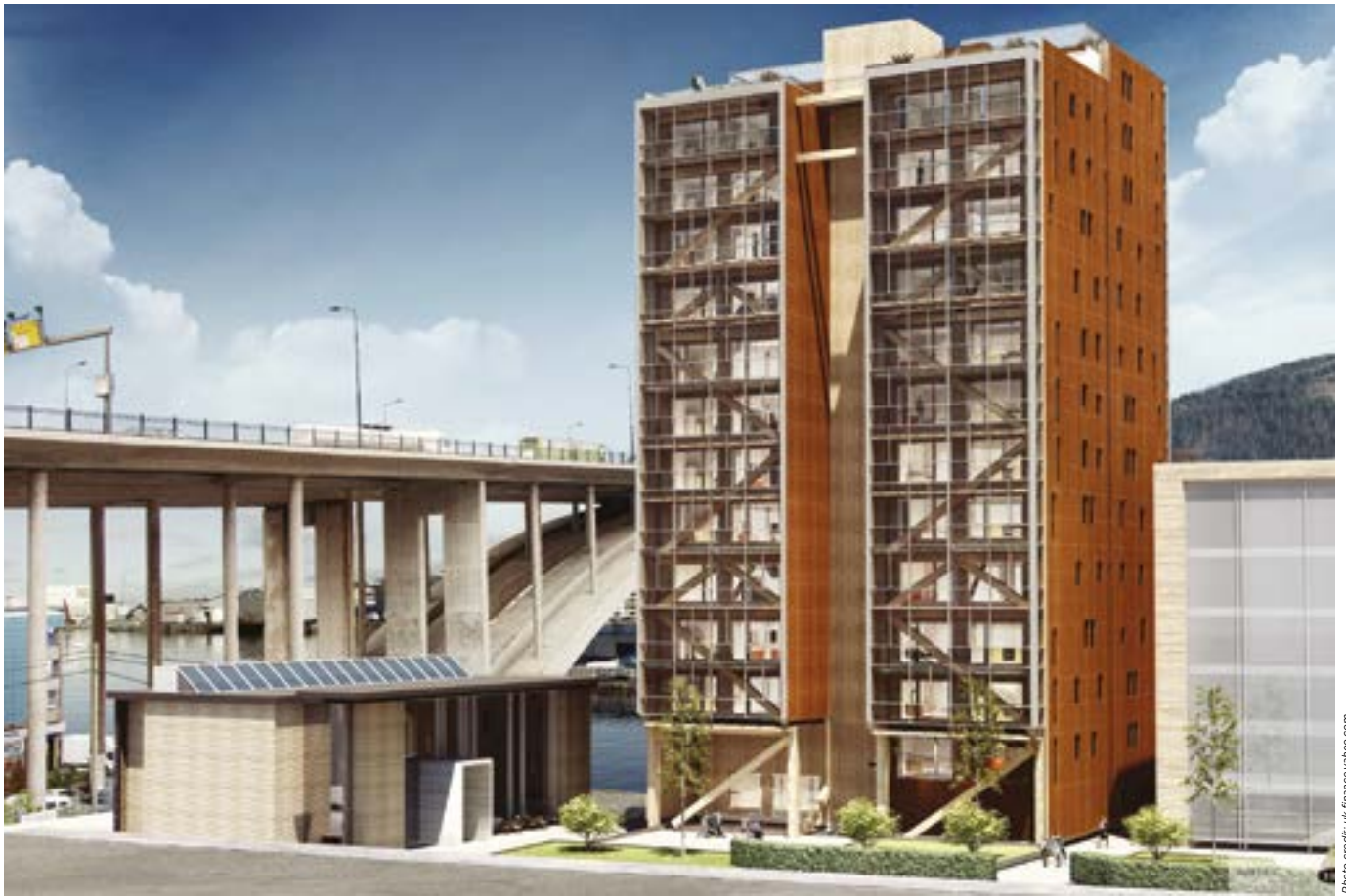
The fire design of TREET is Eurocode-compliant and the glulam used is so thick that it would burn for at least 90 minutes before disintegrating.
