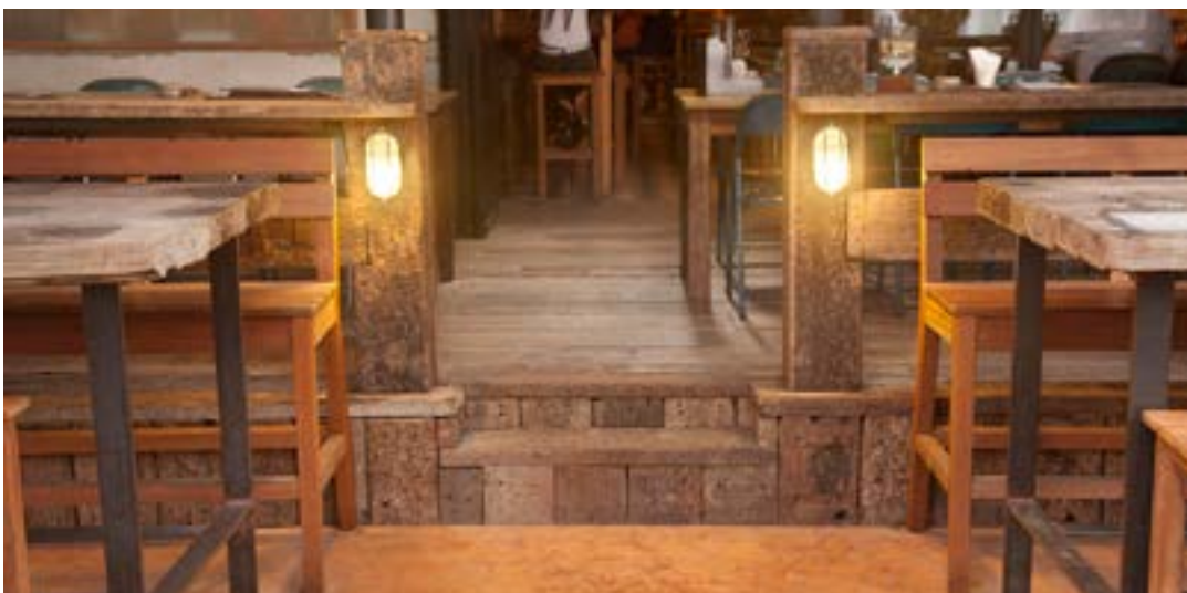
Steps, posts and flooring at the patio are all made from reclaimed Chengal and former railway sleepers.
